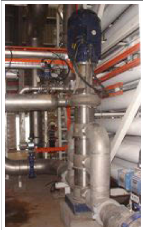
LPH with 3 modules in Singapore
