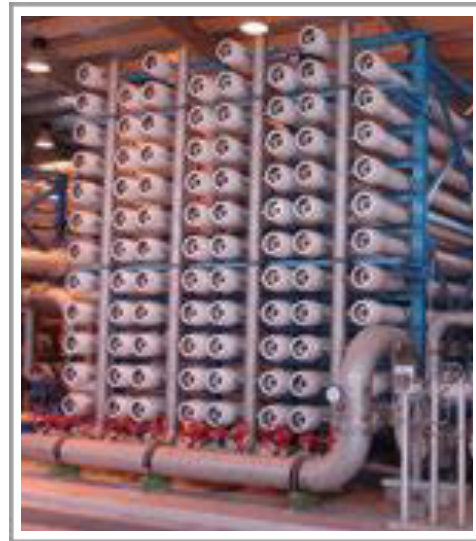
SWRO train with HPB at lower right
